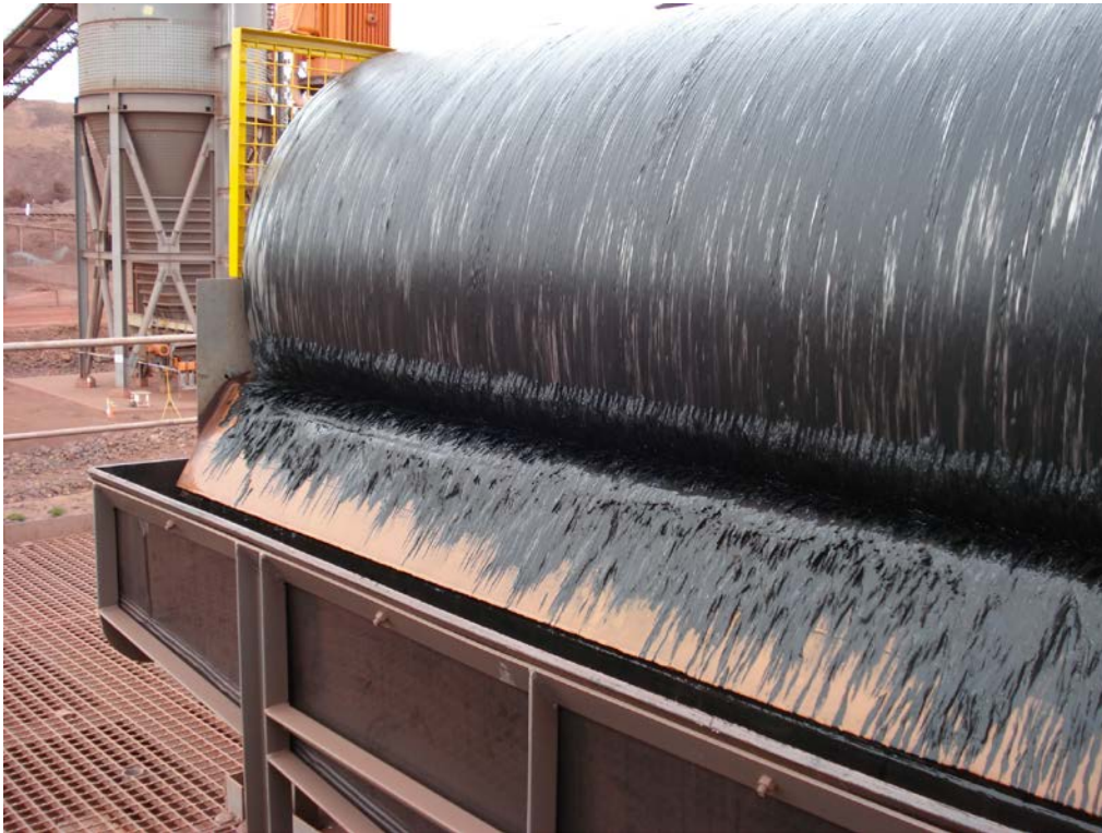
Figure 2: A CMS drum in operation at OneSteel in Whyalla
