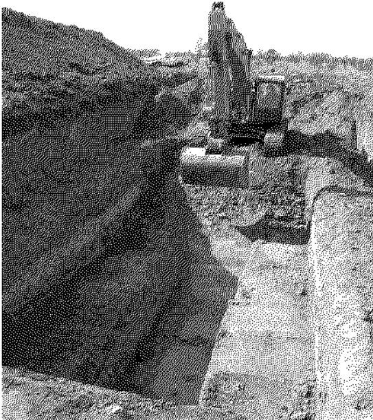
Trench 1 – Excavation. Note stability of walls.
