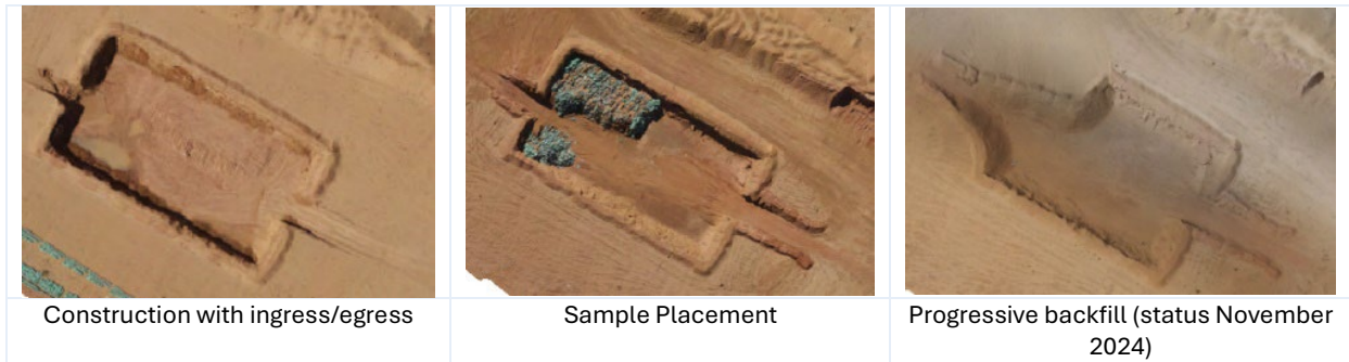
Figure 34: Progressive Backfill of the Sample Disposal Pit
