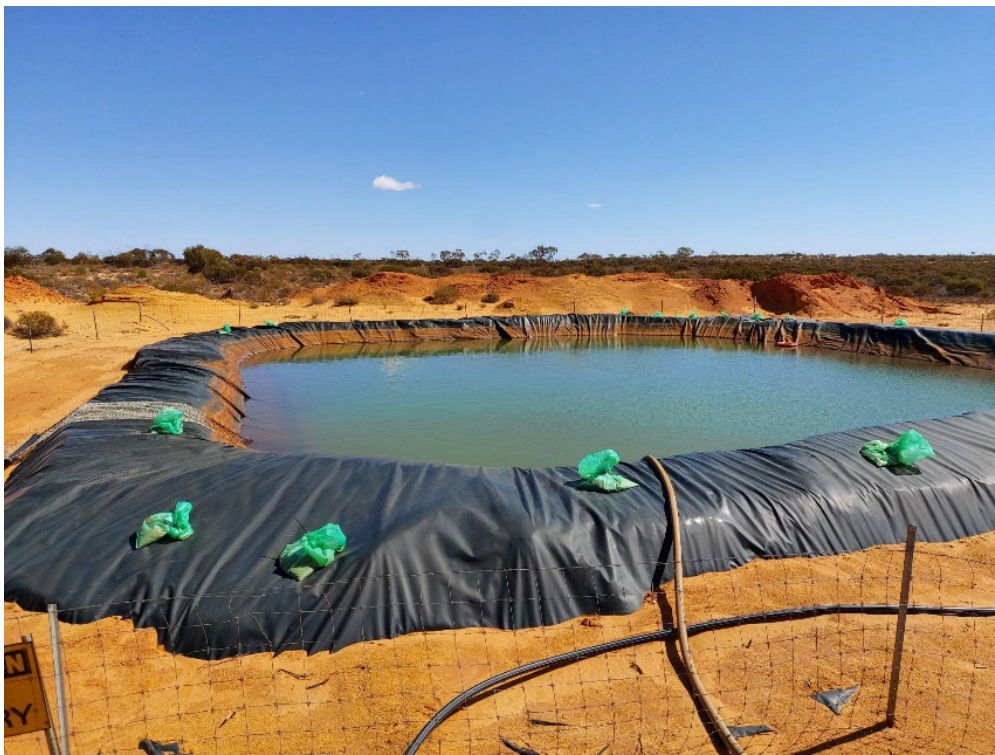
Figure 29: Bore MRWB07 Turkey Nest Facility
