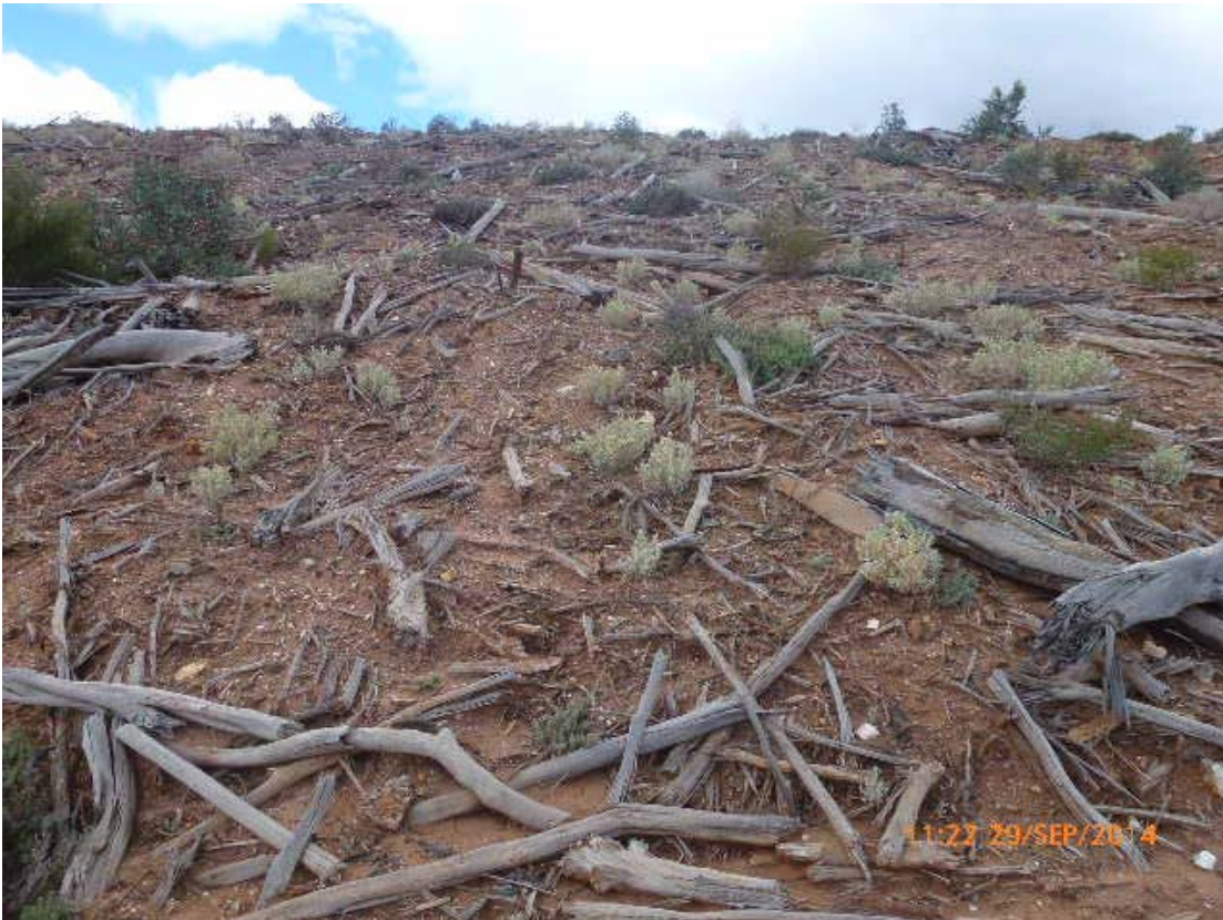
Plate 5.1: Satisfactory utilisation of vegetation debris providing a continuous cover across a slope surface
