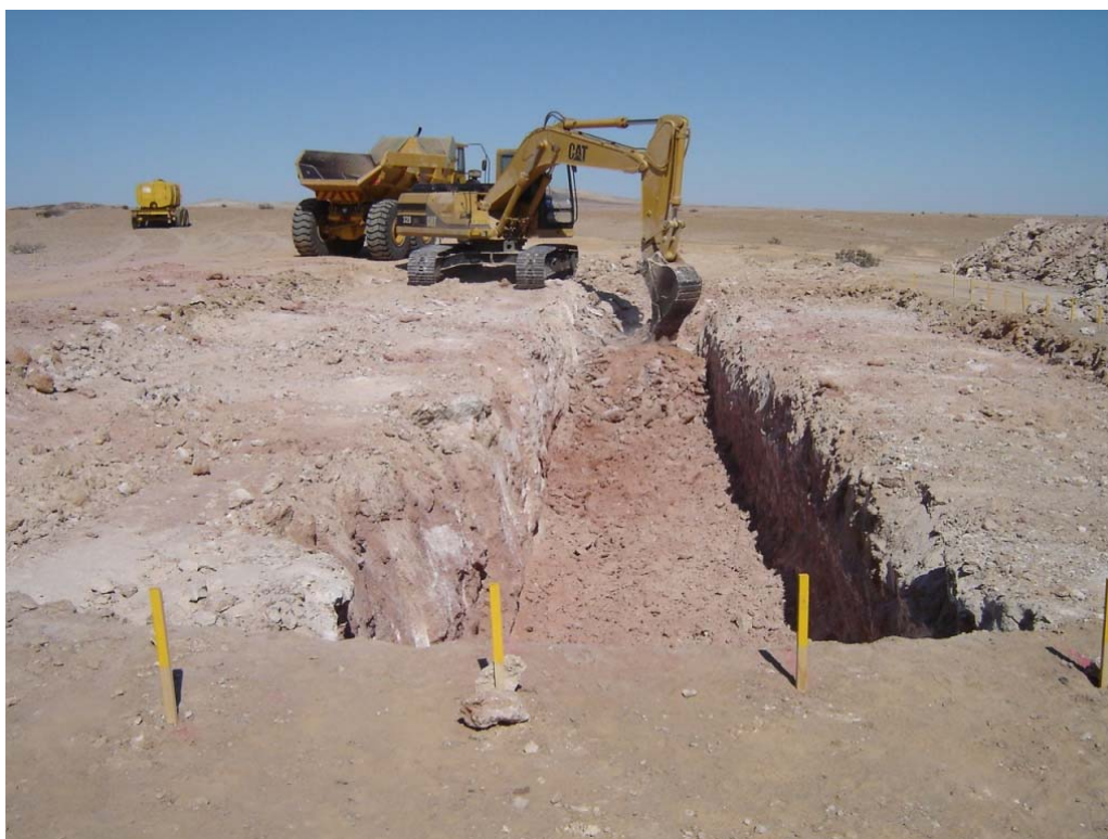
Tubas: Start of trench through surface gypsum layer
