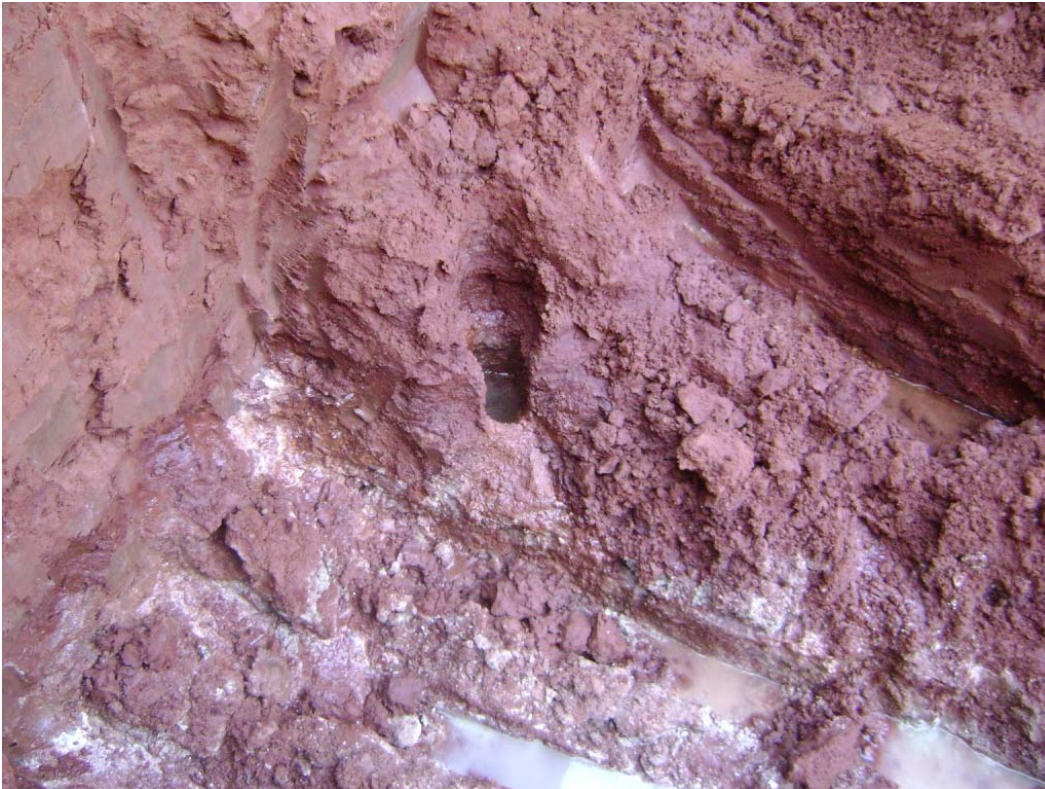
Tubas: Trace of borehole at 10.5 metre
