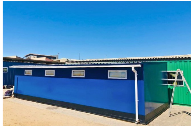
AFTER maintenance work.
