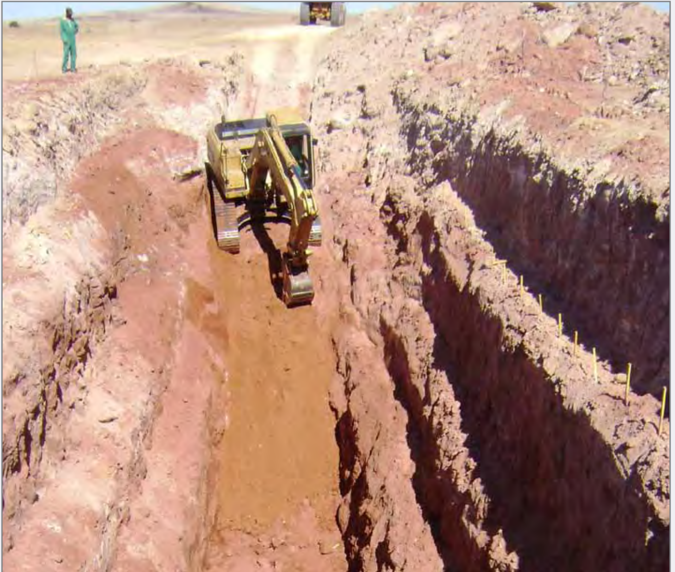
Figure 7: TRS Bulk Sample Trench
