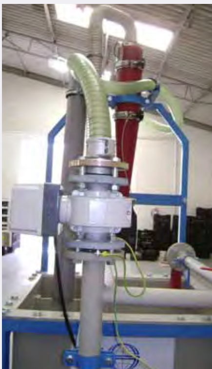
Schauenburg Pilot Plant
