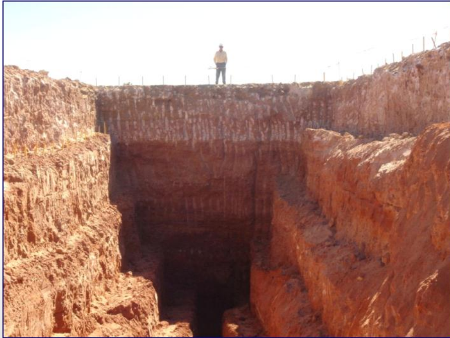
Trench for Bulk Sample
