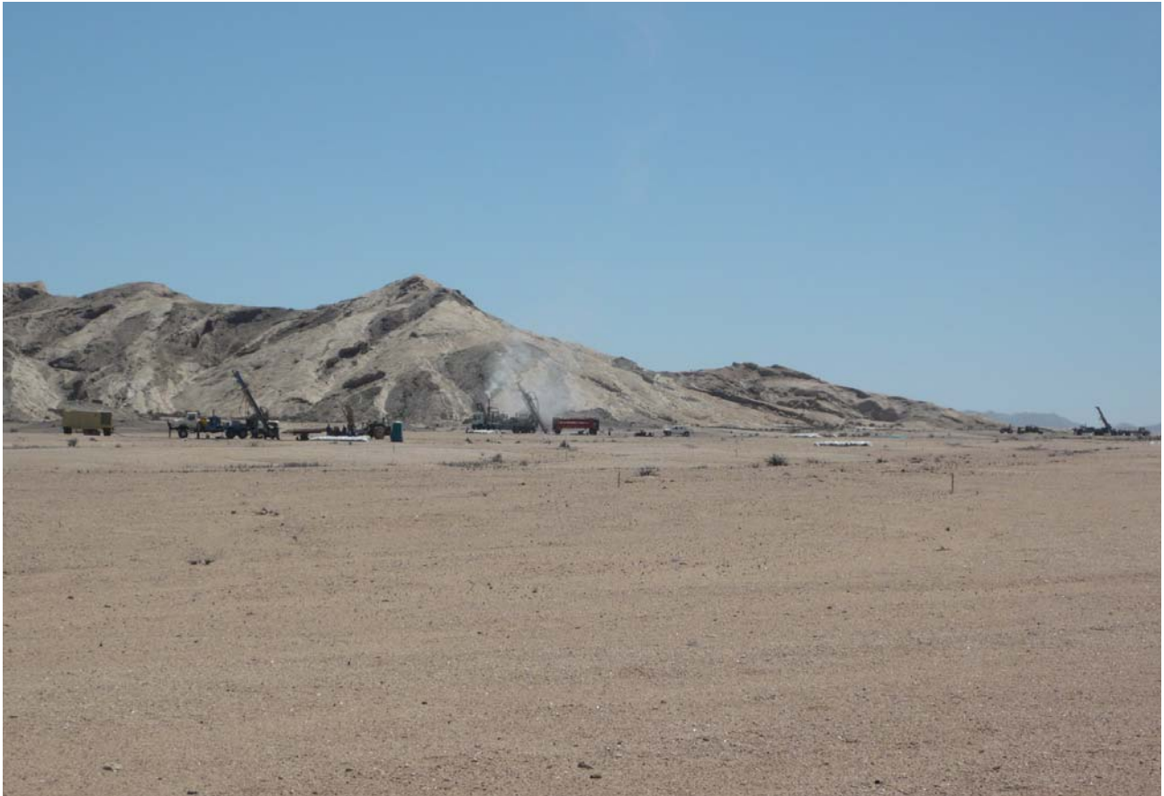
Active Drilling Rigs at the Ongolo Alaskite Project
