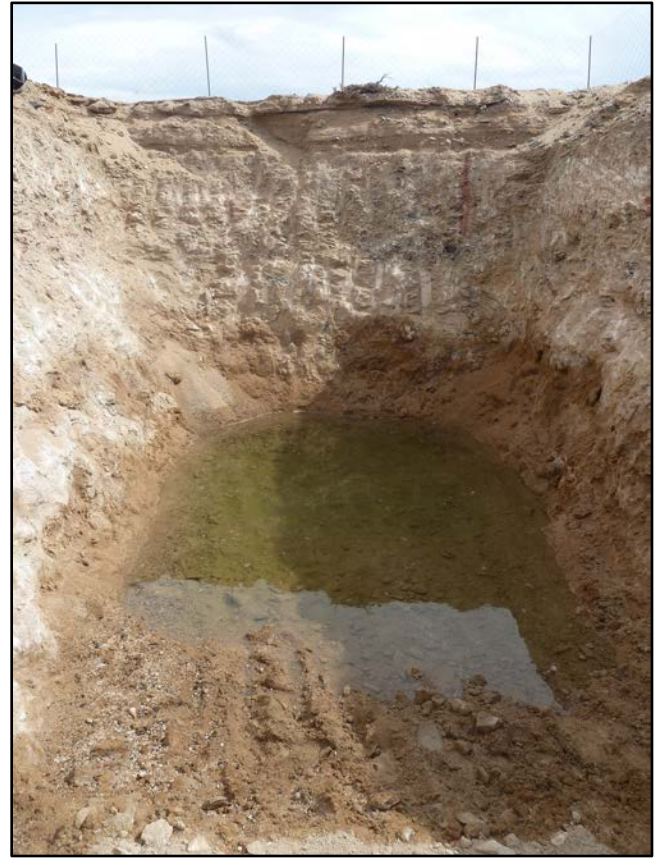
Figure 7. Tumas Trench January 2016
