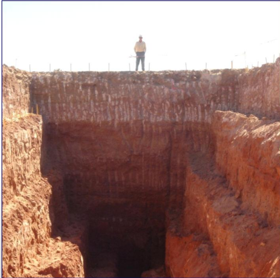
Trench for Bulk Sample
