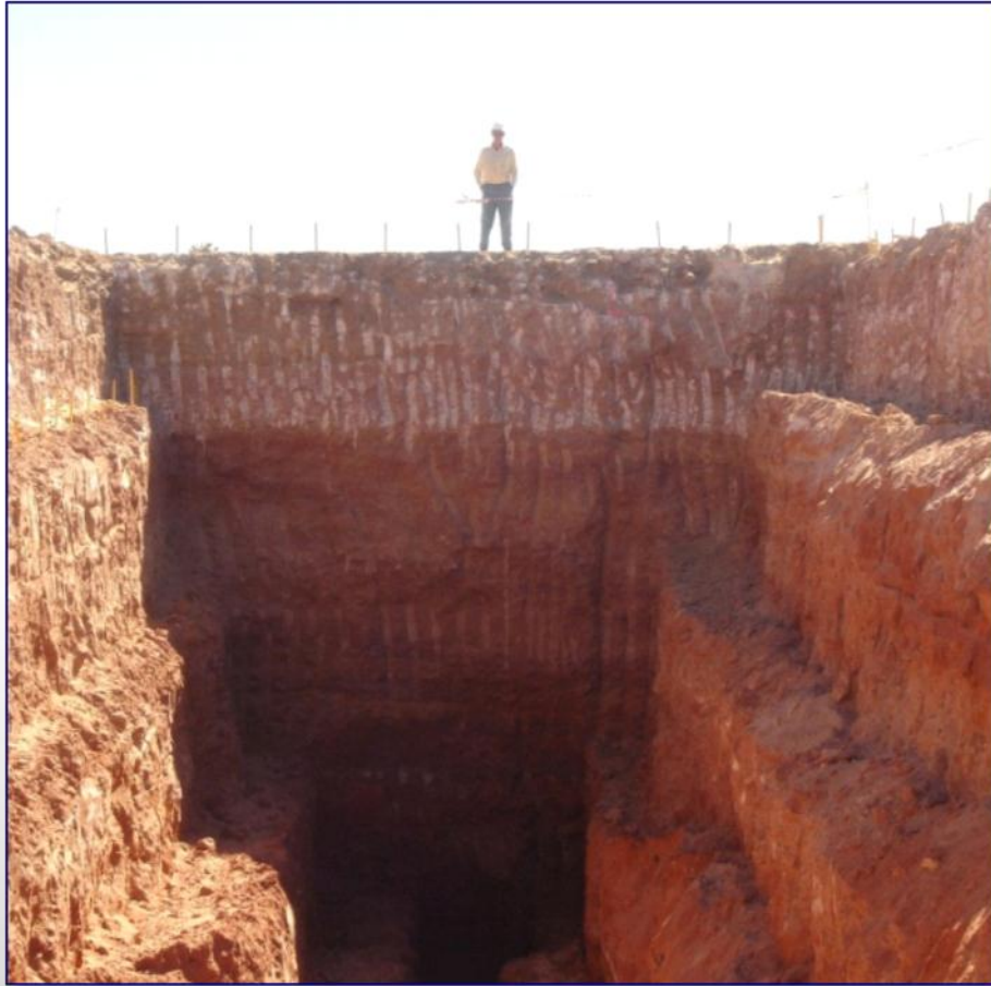
Trench for Bulk Sample
