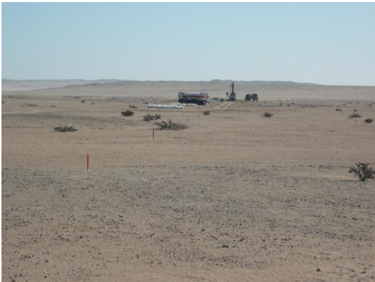
Looking West from Hole SHIR5 to RC Drill Rig on Hole SHIR6 (250 metre)
