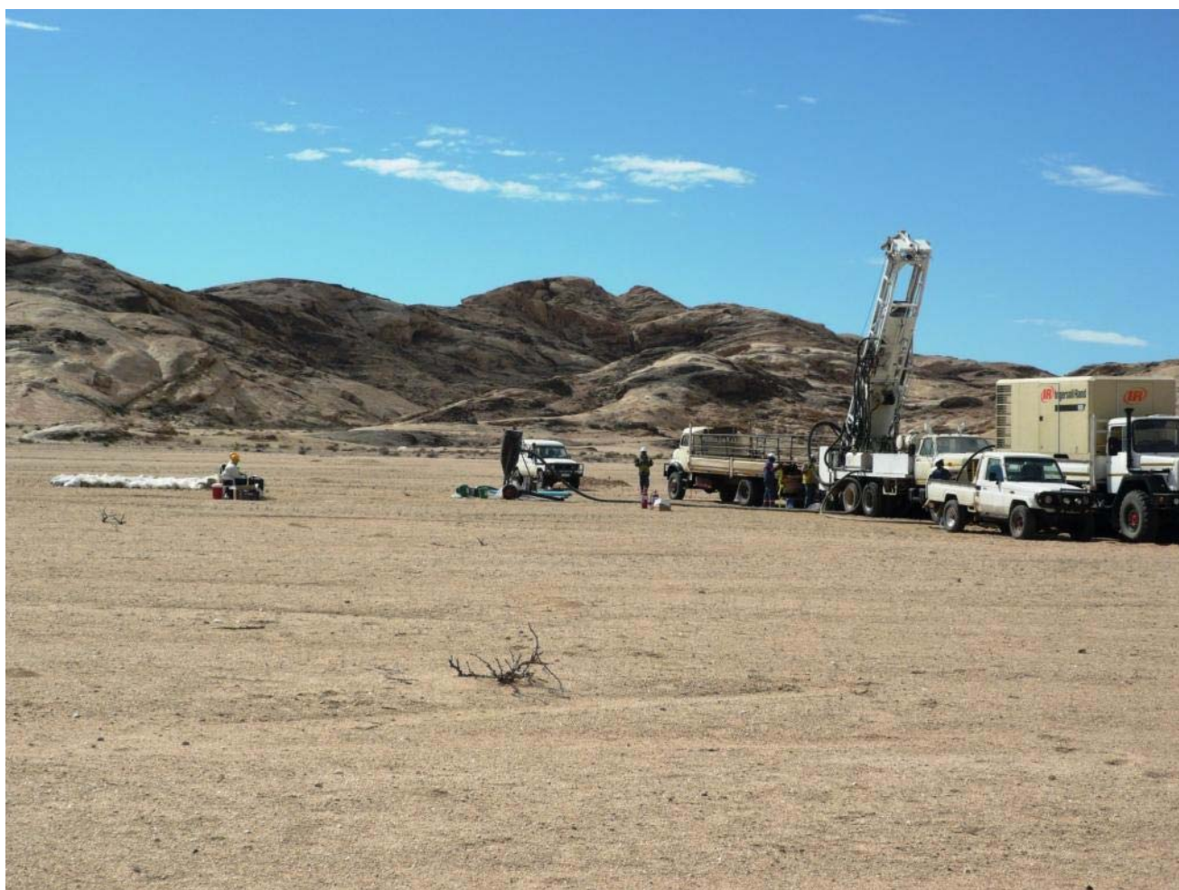
RC Drill Rig at the Tubas Alaskite Project Area
