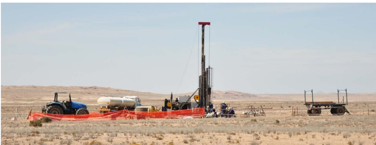
Figure 2: Diamond Drilling for Testwork Core M63 Deposit
