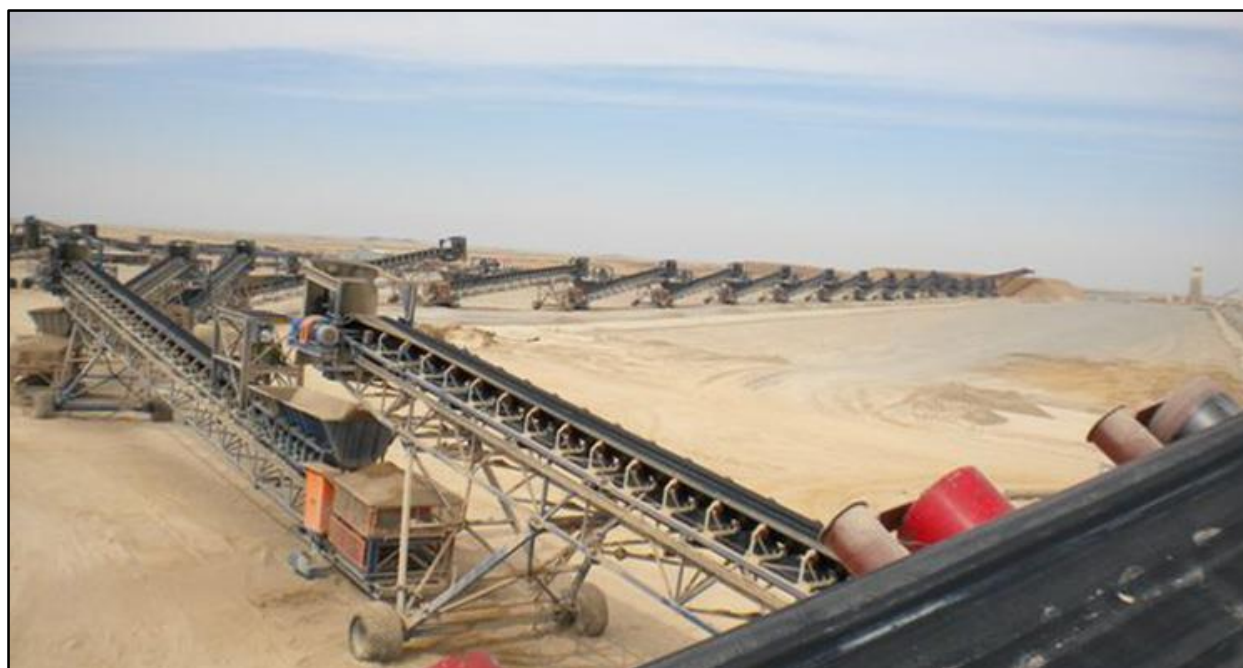
Figure 6: Photo of the Grasshopper system installed by SENET at the Trekopje Mine, Namibia
