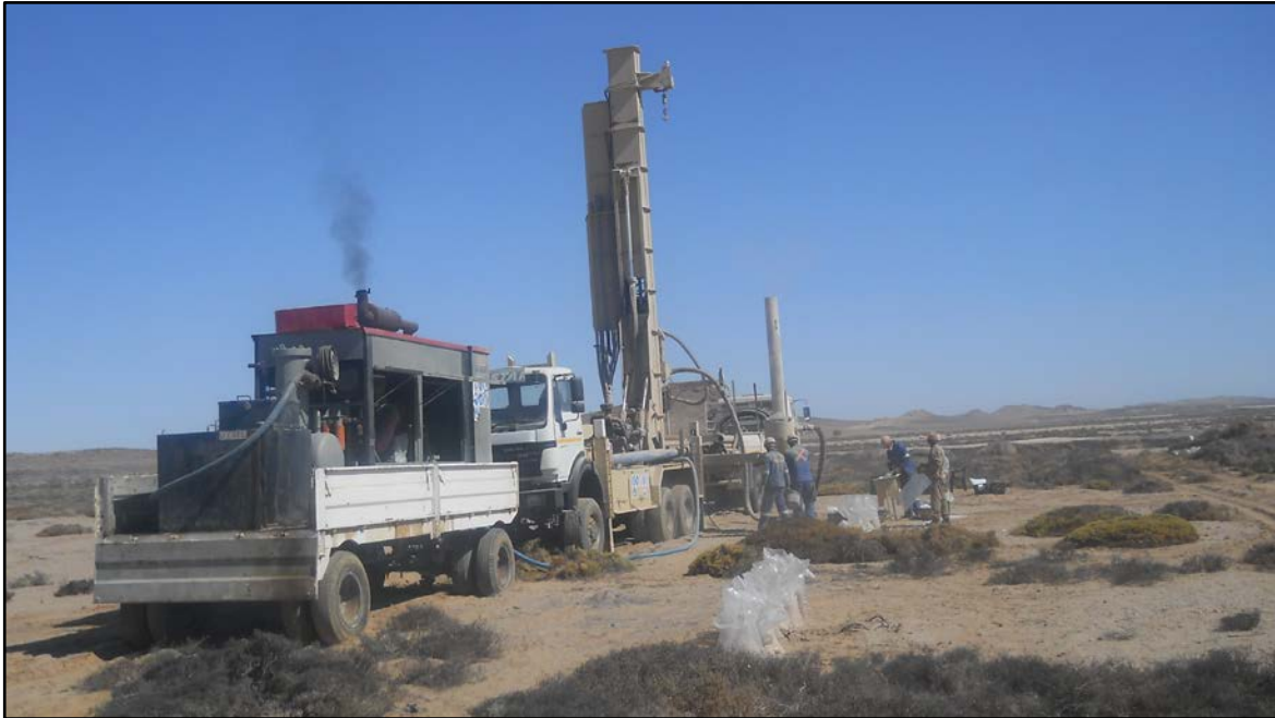
Figure 3: Tumas Project Infill Drilling Campaign, December 2014
