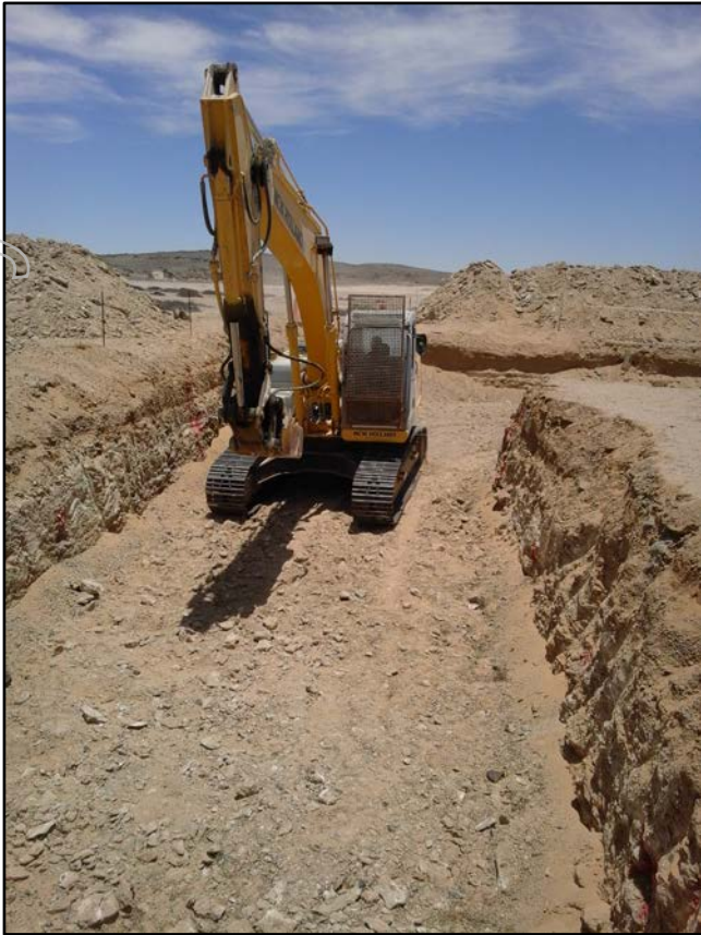
Figure 6. Tumas Excavation December 2015
