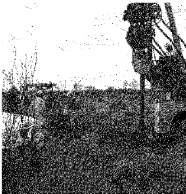
Drilling and sampling above the water table
